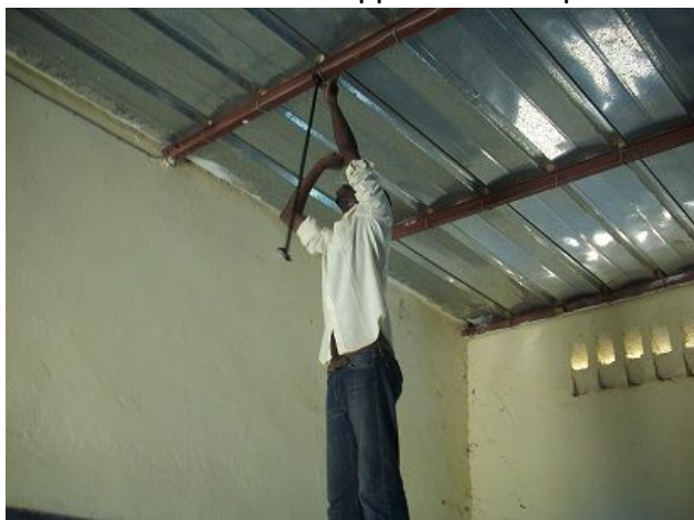
Fixation support de lampe
