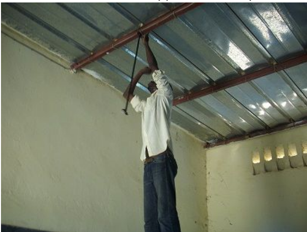
Fixation support de lampe
